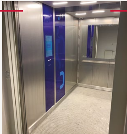
The reconstructed freight elevator in the Z1a building can now be used as a passenger lift as well. And the reconstruction of the second personal elevator has just started.
